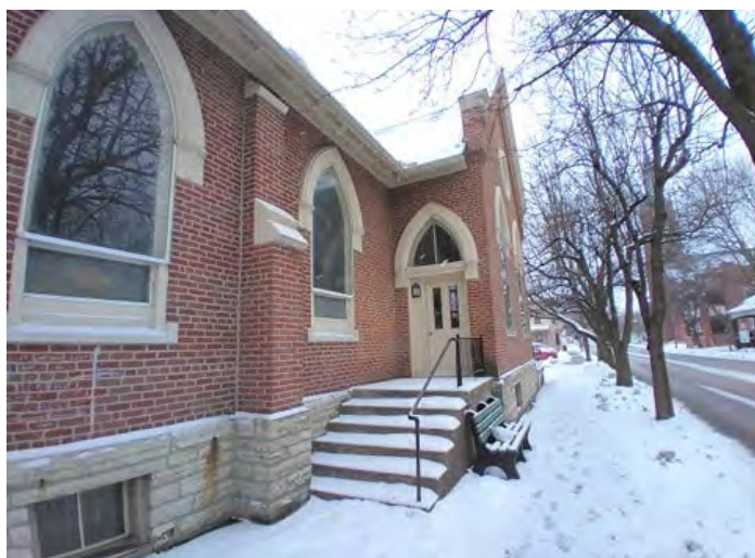
PARTIAL WEST SIDE & NW ENTRY— VIEW SOUTH
