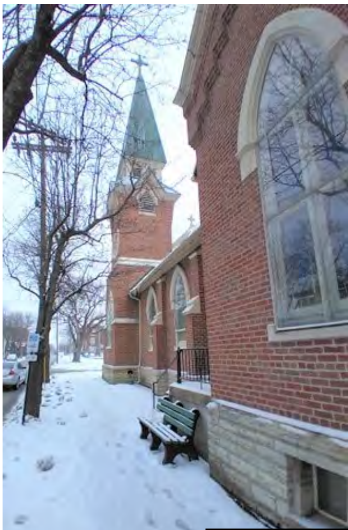
PARTIAL WEST SIDE— VIEWS NORTH
