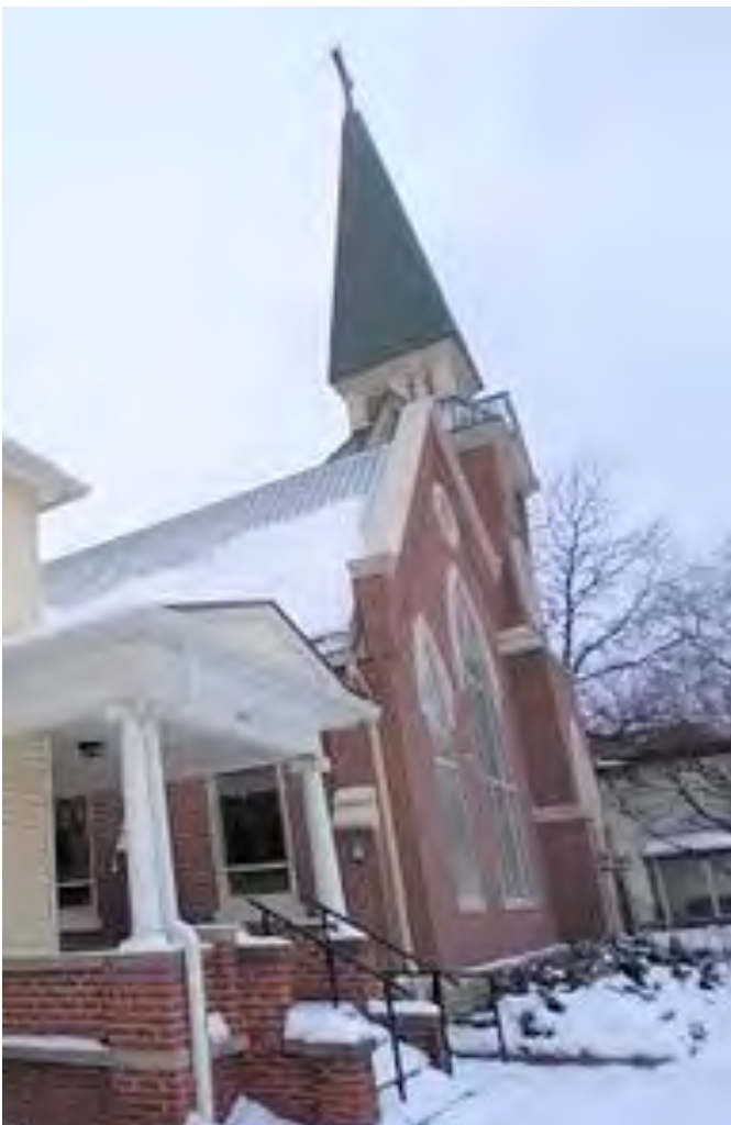
PARTIAL EAST & NORTH SIDES OF CHURCH
